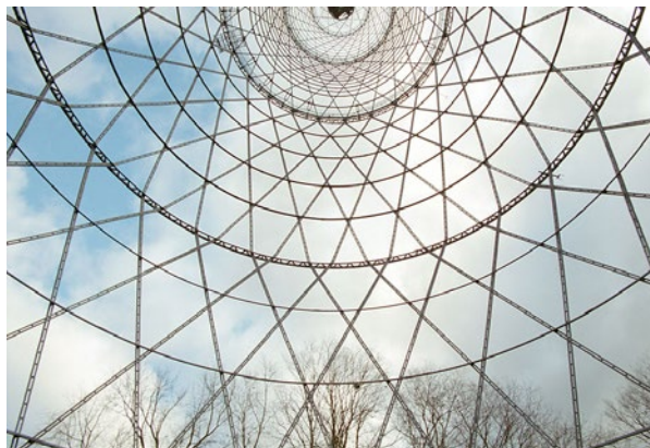
The Shukhov tower is a diagrid structure and an icon of Constructivism, recently spared from demolition.
